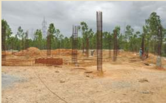
Hospital under construction, Koorgahally
