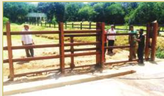
Barricade at African Elephant Enclosure: A new barricade was constructed at African Elephant enclosure using heavy gauge iron railings.
