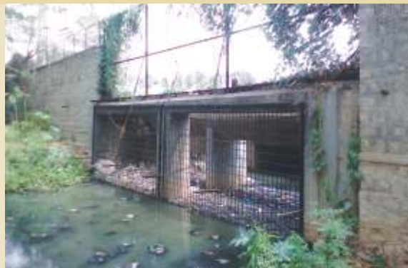
Providing Gates to storm water drain
