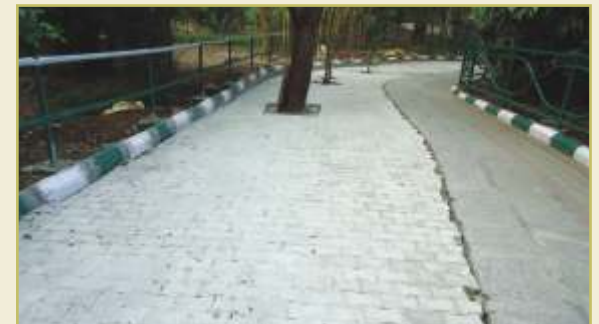
Widening of path between Chimpanzee & Baboon enclosure
