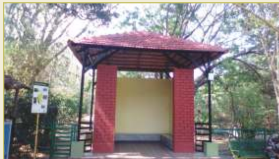
Renovation of rest room near Indian Elephant enclosure
