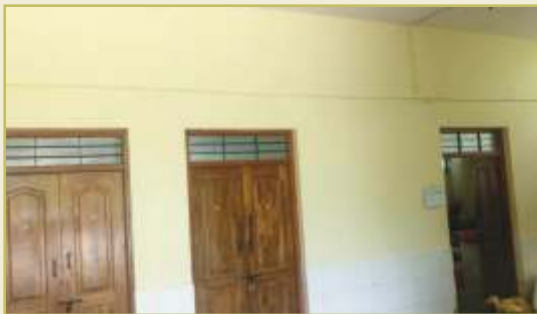
Painting Work at Store
