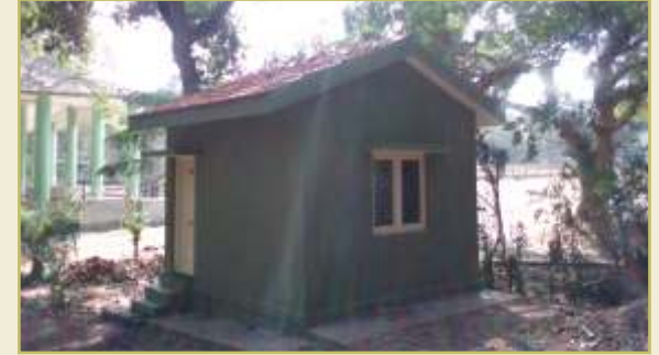
Construction of keepers room near African Elephant enclosure
