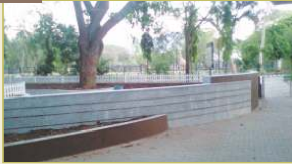
Food court renovation at Amphitheatre
