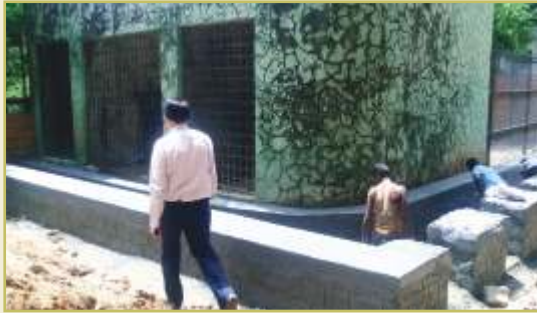
Drain at Neelghai Enclosure: Whenever there is heavy rain due to improper drainage water stagnation at the end of Neelgai enclosure is used to be a common problem. The drainage was constructed to facilitate the flow of rain water & the problem was resolved.
