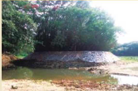
Karanji island revetment
