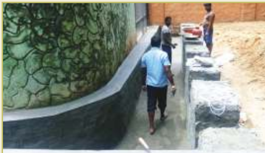
Drain at Neelghai Enclosure: Whenever there is heavy rain due to improper drainage water stagnation at the end of Neelgai enclosure is used to be a common problem. The drainage was constructed to facilitate the flow of rain water & the problem was resolved.
