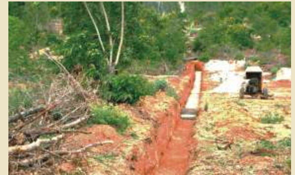
Gaur enclosure under construction
