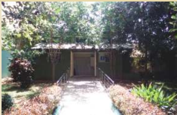
Renovation of Toilets
