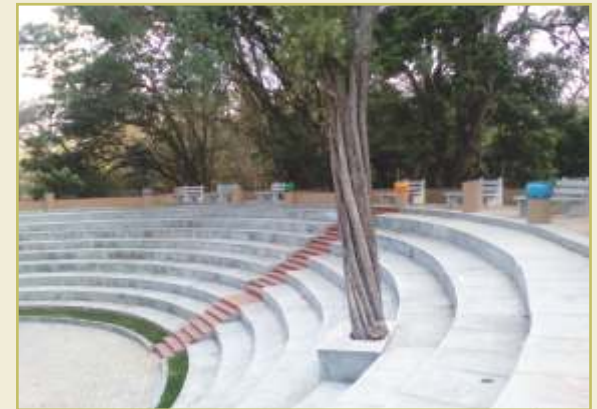
Land scaping works made in Amphitheatre Steps in Amphitheatre
