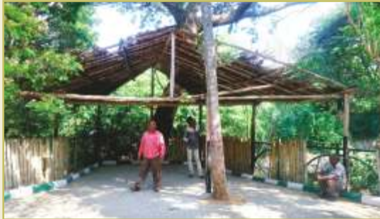
Visitors shelters made out of thatched roofs using coconut palms
