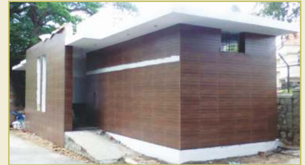
Construction of rest room at Giraffe Enclosure
