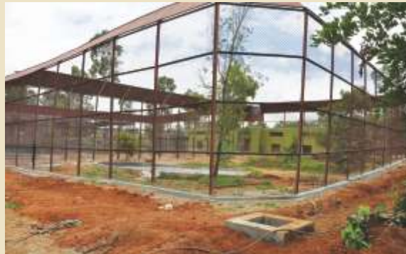
construction of day kraal
